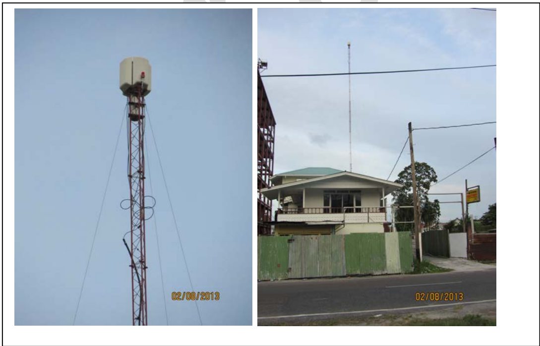
Figure 3 Typical TV transmitter in Georgetown
